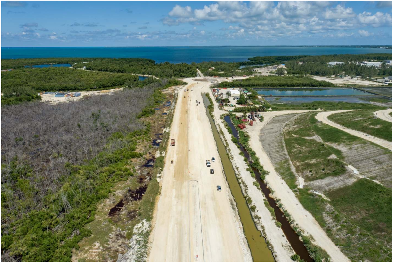
Base Layer being prepped for paving in October
