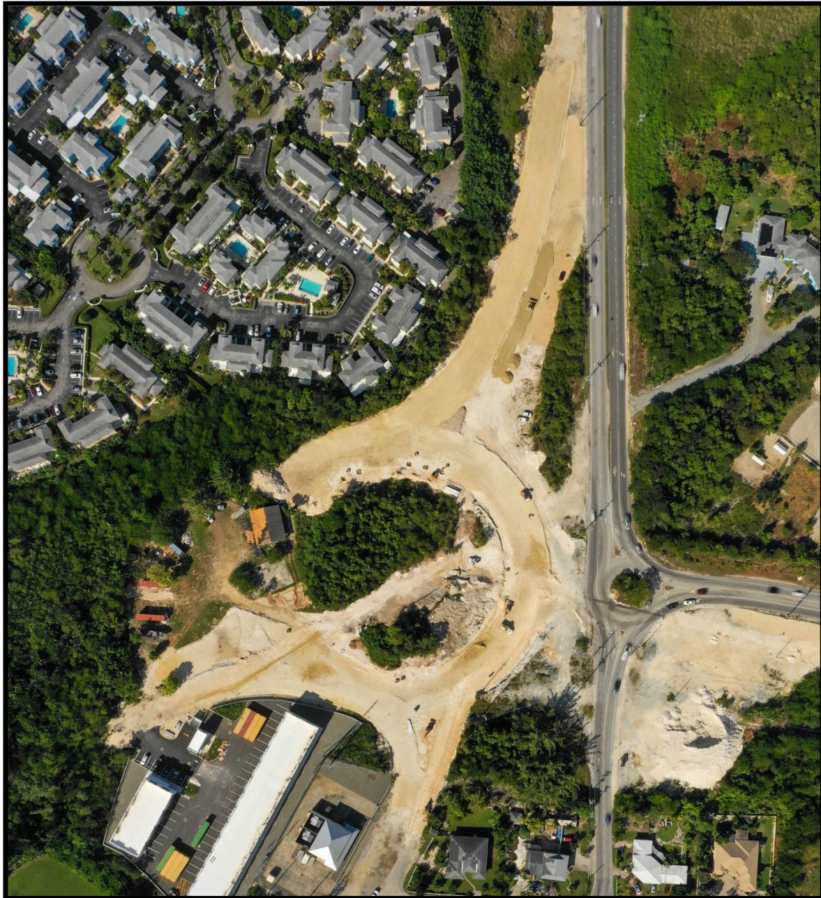
Linford Pierson Highway/Bobby Thompson Way Roundabout taking shape
