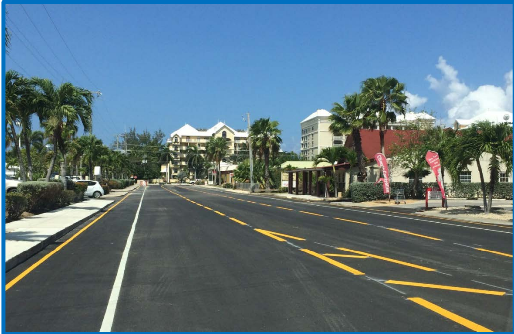
Road Surface Upgrades at Canal Point Road at The Strand Complex
