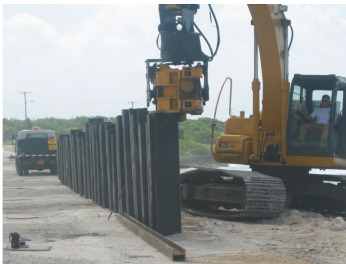
Steel Sheetpiles being hammered into bedrock – Clarinda Beach East End
