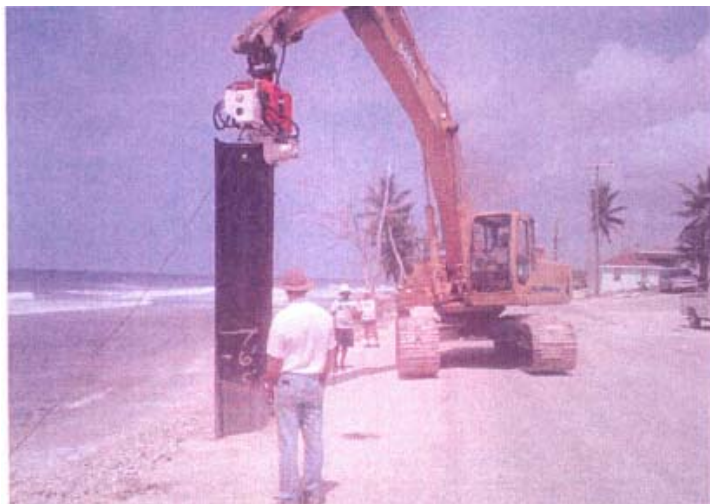
June 2007 – engineers install test piles at LEB seawall site
