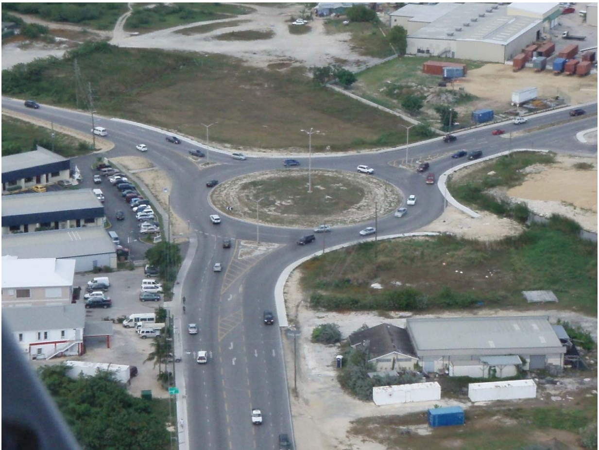
Aerial view of new roundabout on Elgin Avenue
