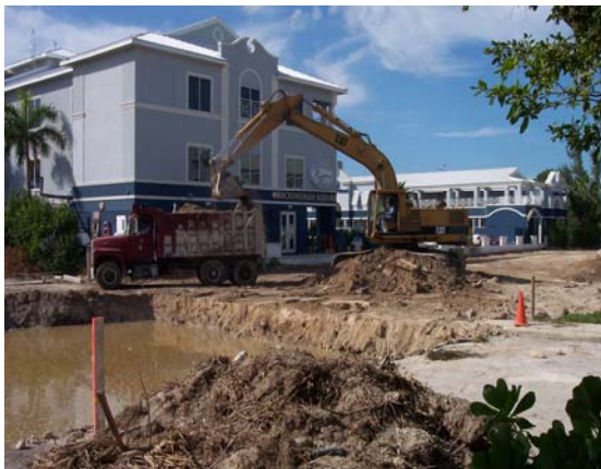
Demucking on section of ETH by Buckingham Place Feb06
