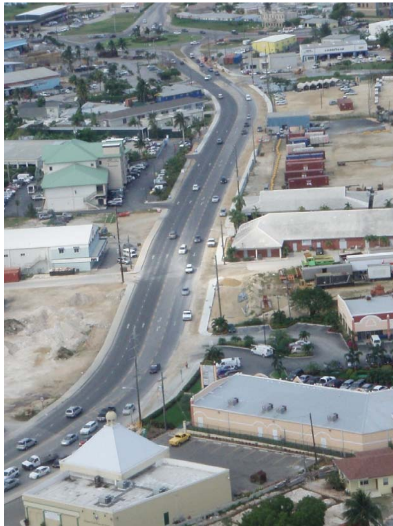
Aerial view of new ETH & LPH connector
