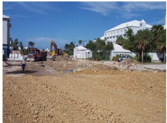
Installation of road base material on ETH
