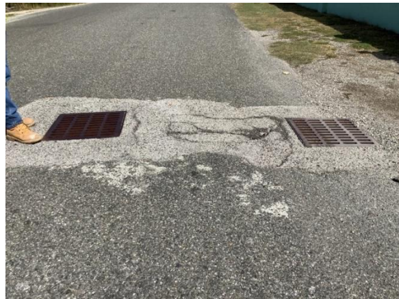
Figure 12-12: Inlet on Shoulder Drains to Inlet in Centre of Roadway (July 2023)
