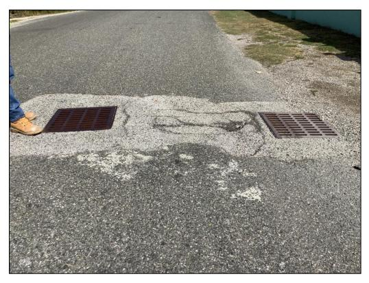
Photo 6: Inlet on shoulder drains to inlet in centre of roadway (July 2023)
