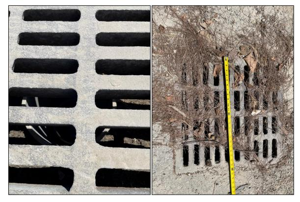
Photo 9: Inlet clogged with sediment (top) and debris (bottom) (July 2023)
