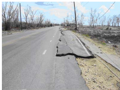
(Left) Strong storm surge and battering waves removed a section of the asphalt along South Sound Road. (Right) Spotts Straight, along Shamrock Road, shows damage from storm surge during Ivan.
