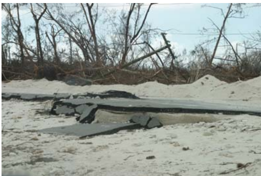
(Left) Strong storm surge and battering waves removed a section of the asphalt along South Sound Road. (Right) Spotts Straight, along Shamrock Road, shows damage from storm surge during Ivan.
