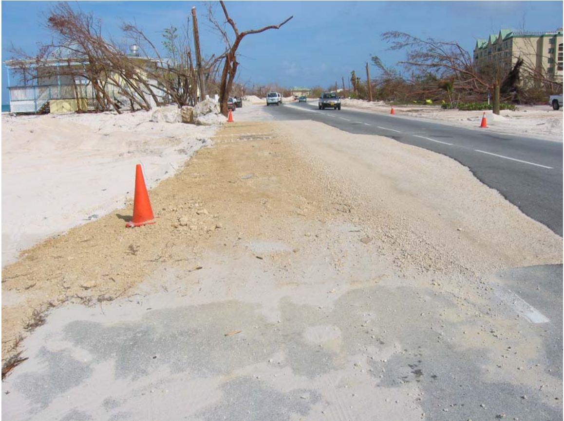
Emergency Patch – installed by NRA pending permanent repair work
