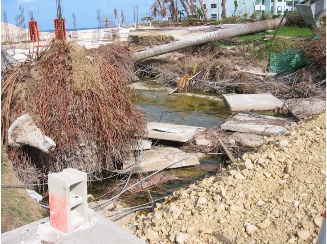
West Bay Road – Sink Hole North of Canal Point
